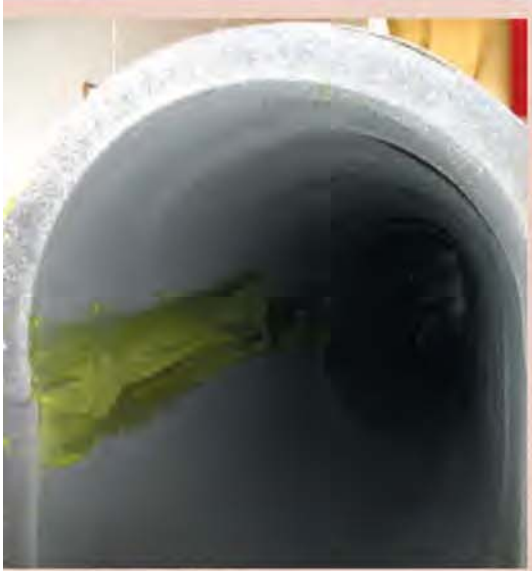
A close-up of the K-Flex elastomeric installation inside the duct.
